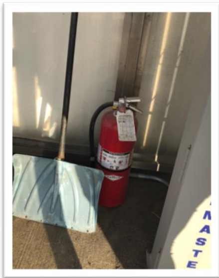
L-R: an unmounted fire extinguisher, congestion around an emergency exit, and storage in front of fire extinguisher
